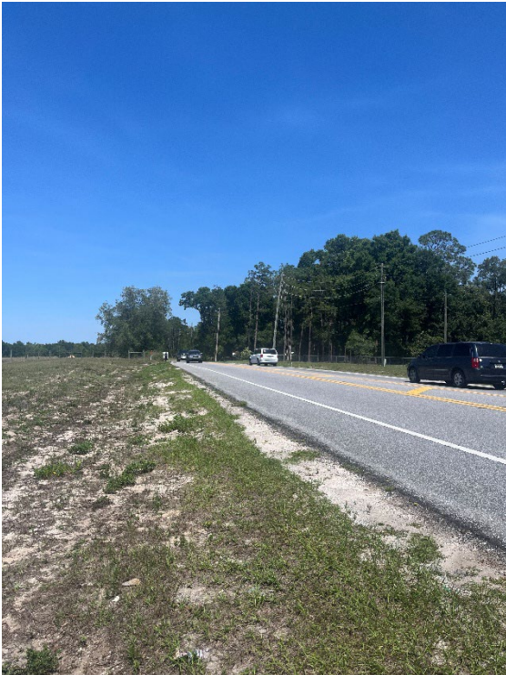
Looking east on SE 110 th Street Rd.
