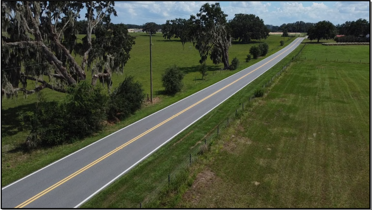
View looking south along SE 73rd Ave
