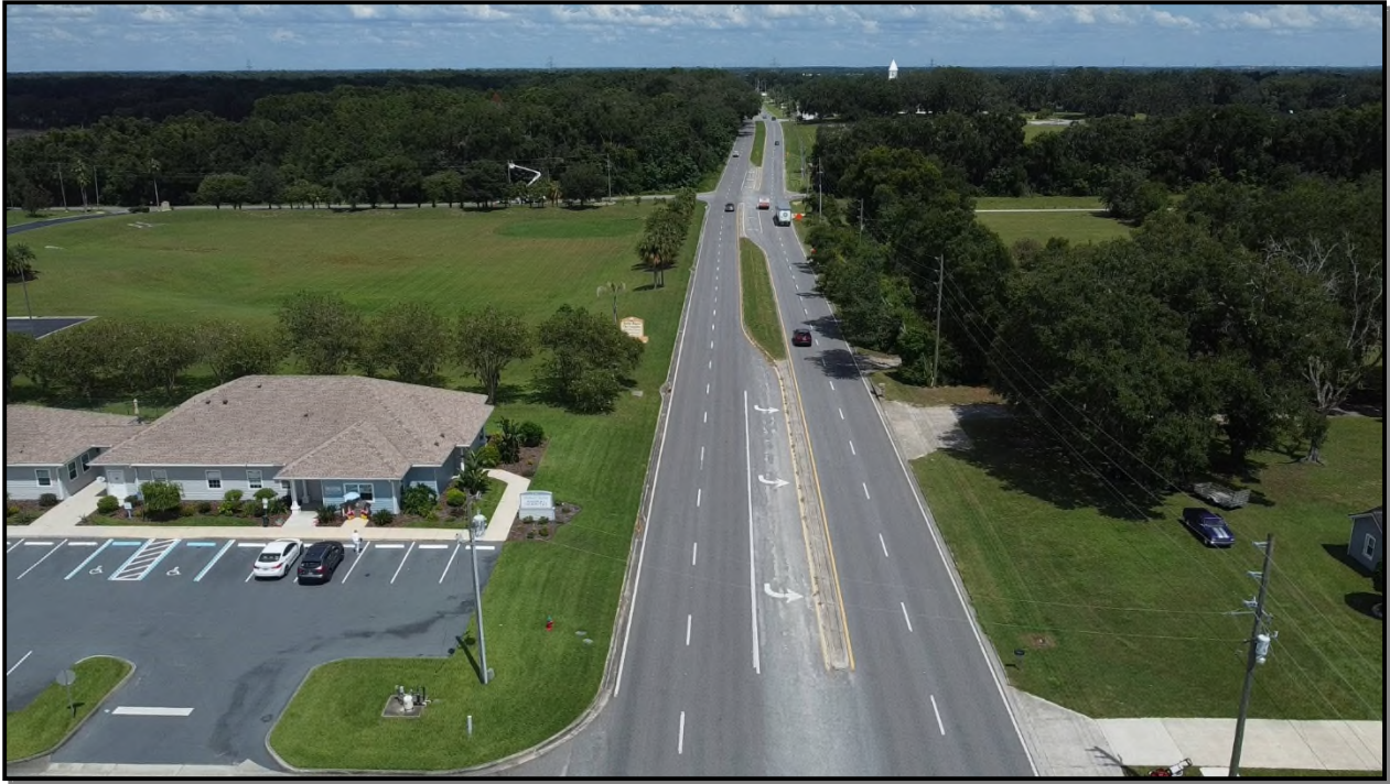
View east along SE County Road 42
