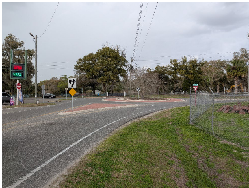
Figure 15. View of roundabout at intersection of NE 97 th Street Road and NE 21 st Avenue
