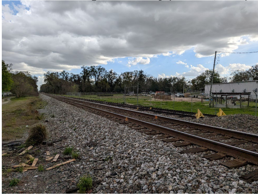
Figure 16. View of existing CSX railway (March 6, 2026)
