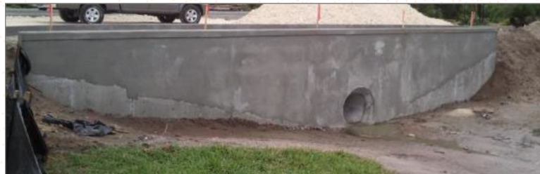
Cantilever Retaining Wall
