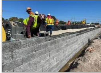
Segmental Block Wall
