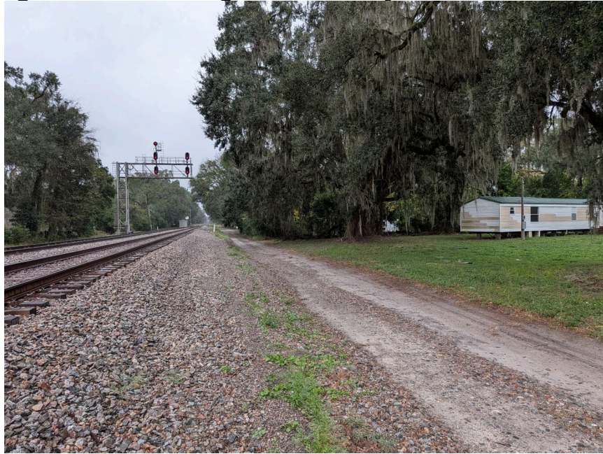
Figure 6. Facing northeast along CSW railway/SE 70 th Avenue Road
