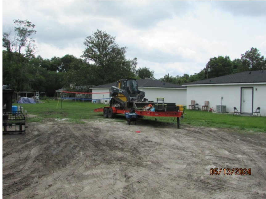
Figure 17. View of material and equipment storage (Code Case No. 934739, 934740, 934741, and 934742)
