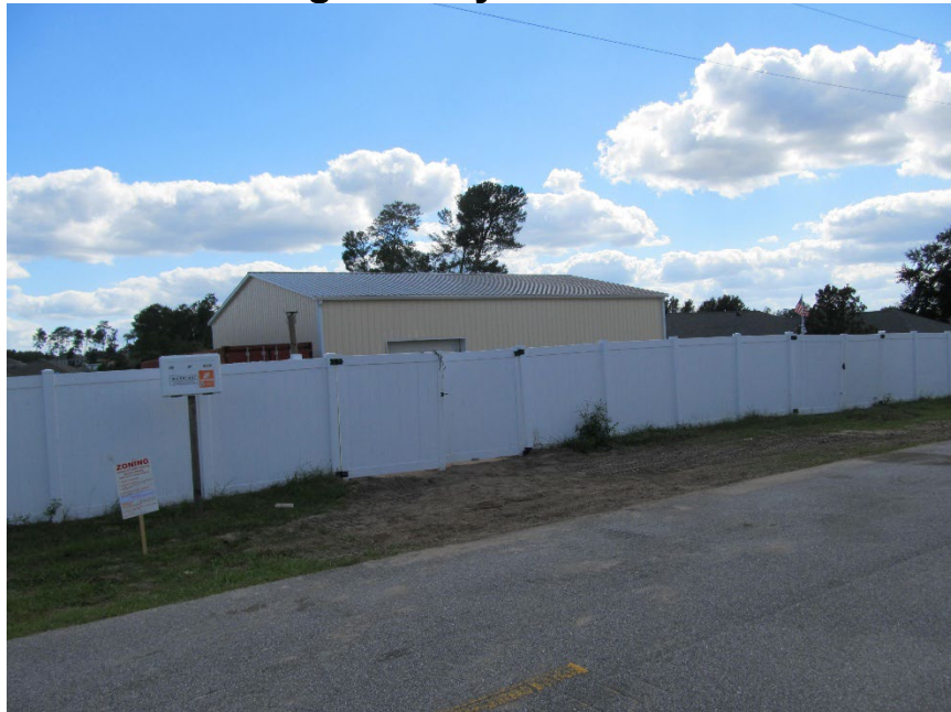
Figure 5. View of storage facility from SW 103 rd Street
