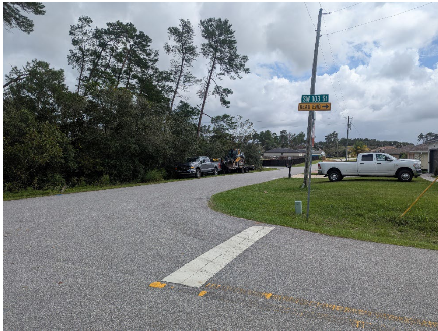
Figure 11. View of flatbed trailer and work vehicle on SW 42 nd Avenue
