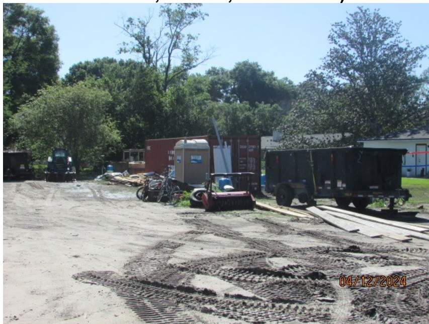
Figure 15. View of material and equipment storage (Code Case No. 934739, 934740, 934741, and 934742)
