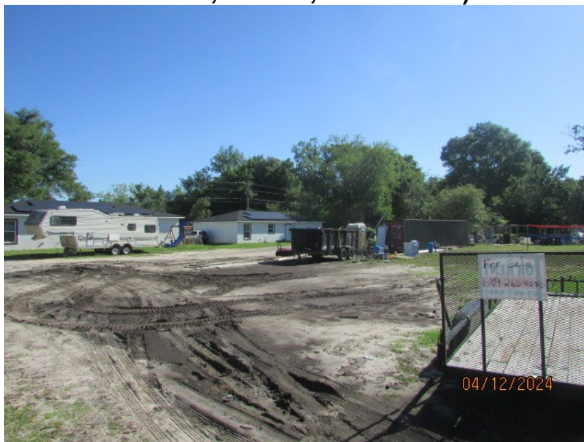
Figure 16. View of material and equipment storage (Code Case No. 934739, 934740, 934741, and 934742)
