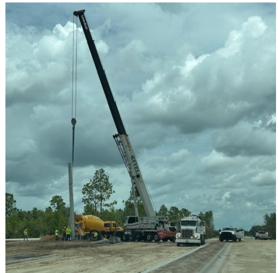
SW 49th Ave Segment F – Signal Pole Installation
