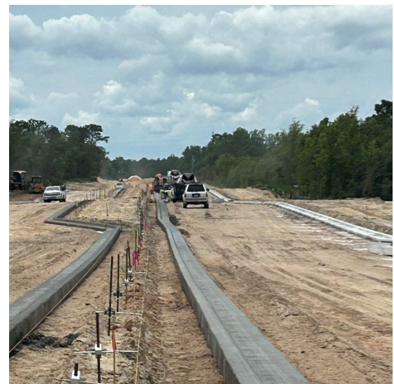
SW 49th Ave Segment F – Curb and Gutter Installation
