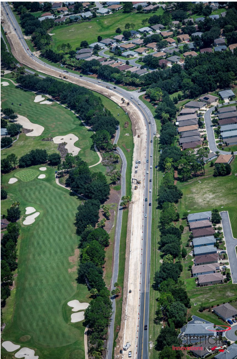
SW 80th Ave Segment 1 Phase A – Looking North along Project
