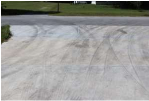
Improved driveway on SW 15 th Place
