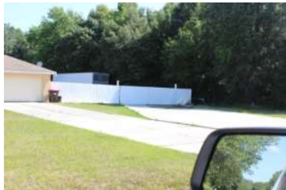
Screening of parking area from SW 15 th Place
