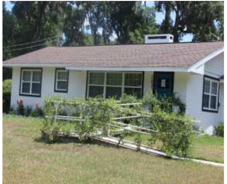
Building on subject property, used for professional office
