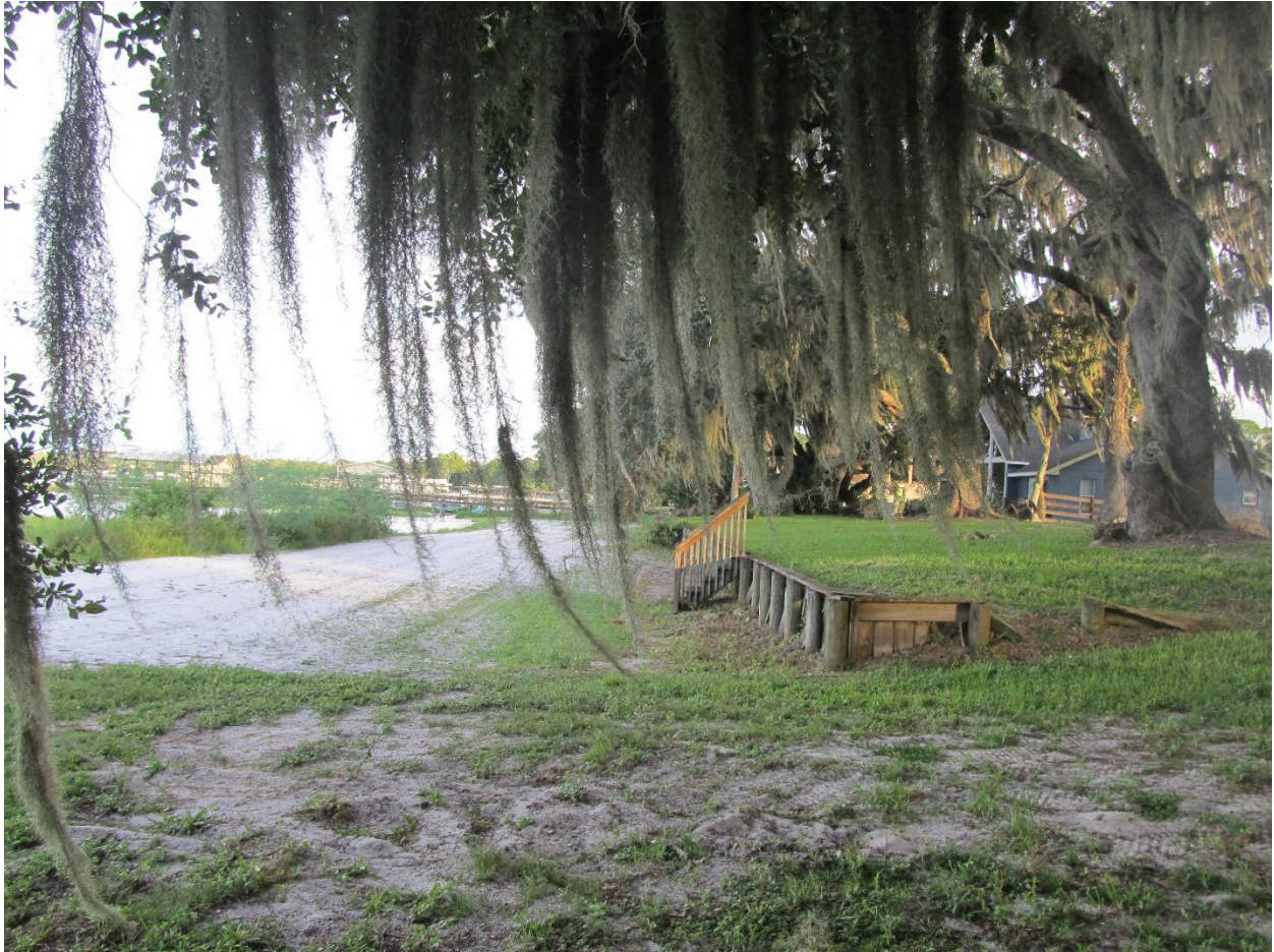
Looking west from east property line at seawall. Water to the left.
