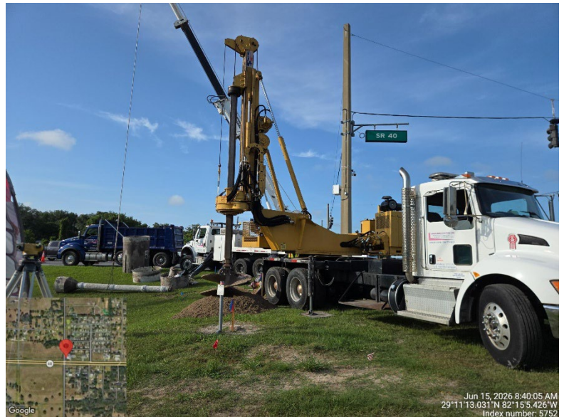
SR 40 at NW/SW 80th Ave Intersection – Drilled Shaft Installation
