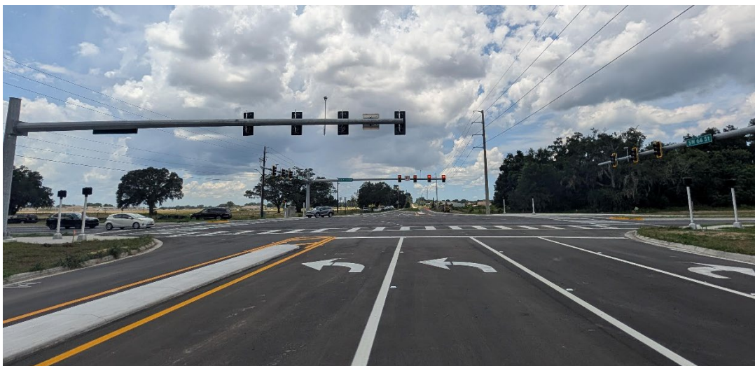
SW 49th/40th Ave Phase 1 – Signal at SW 66th St Intersection
