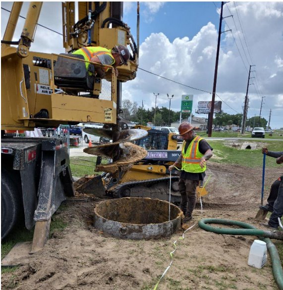
SR 40 at NW/SW 80th Ave Intersection – Drilled Shaft Installation
