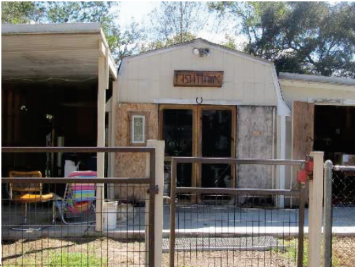
3. View of distillery building.
