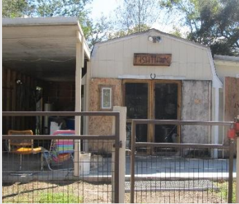
View of distillery building.
