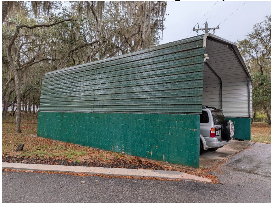
Figure 7. Alternative view of existing RV carport
