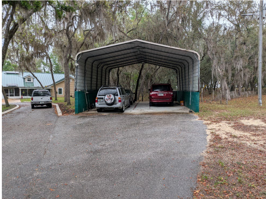
Figure 6. View of existing RV carport
