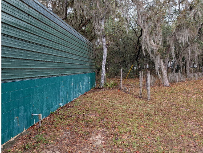
Figure 8. View of fence adjacent to existing RV carport
