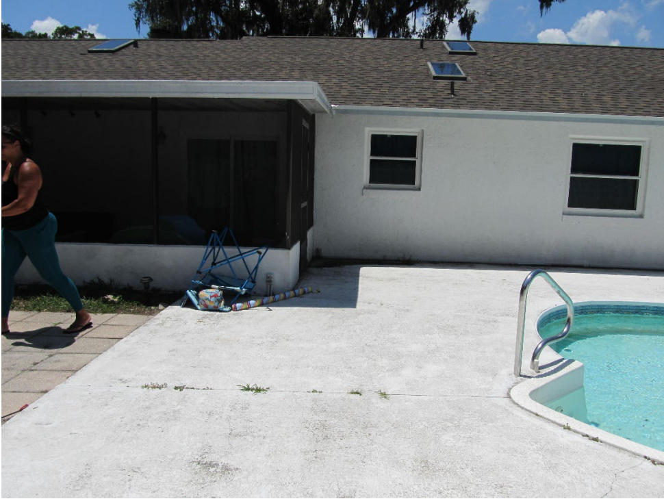
Eastern edge of pool deck at fence line looking west
