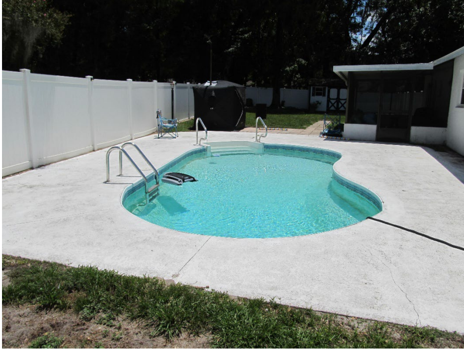
North side of pool decking looking south
